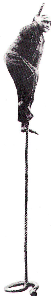
Fig.10.6: The legendary Indian rope trick. The rope stands erect on the ground and a person climbs over it as if he is climbing over a tree.
